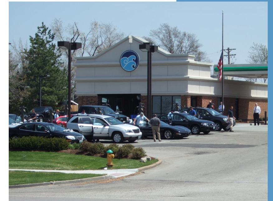
Waterway recently completed a number of renovations to its Chesterfield location.
